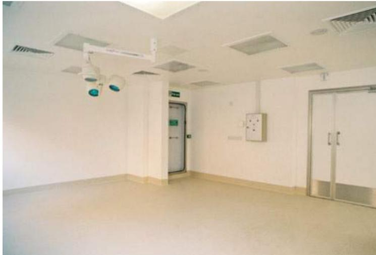
Prior to the application of the coating system, new plasterwork was treated and previously painted surfaces were sealed. The work, carried out while the hospital was still open to patients and the public, involved spraying the Tretoplast WB system on to walls and ceilings of the new theatre and all of its ancillary rooms.
